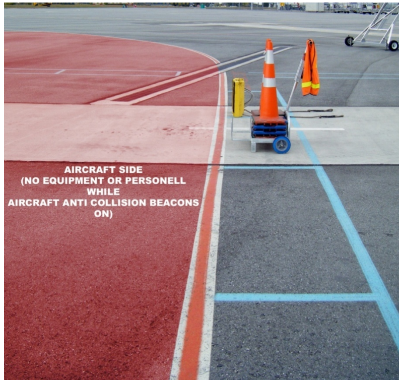
16-6 - Equipment Storage Limit Line
