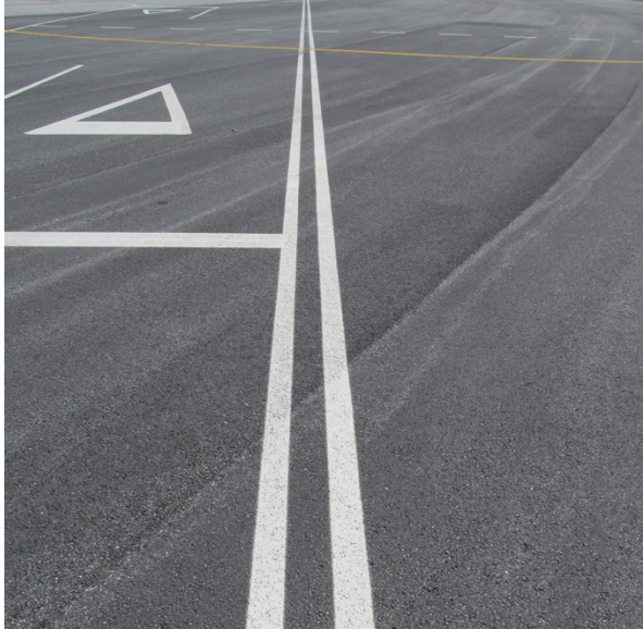
16-12 – Demarcation between apron service road and apron taxiway
